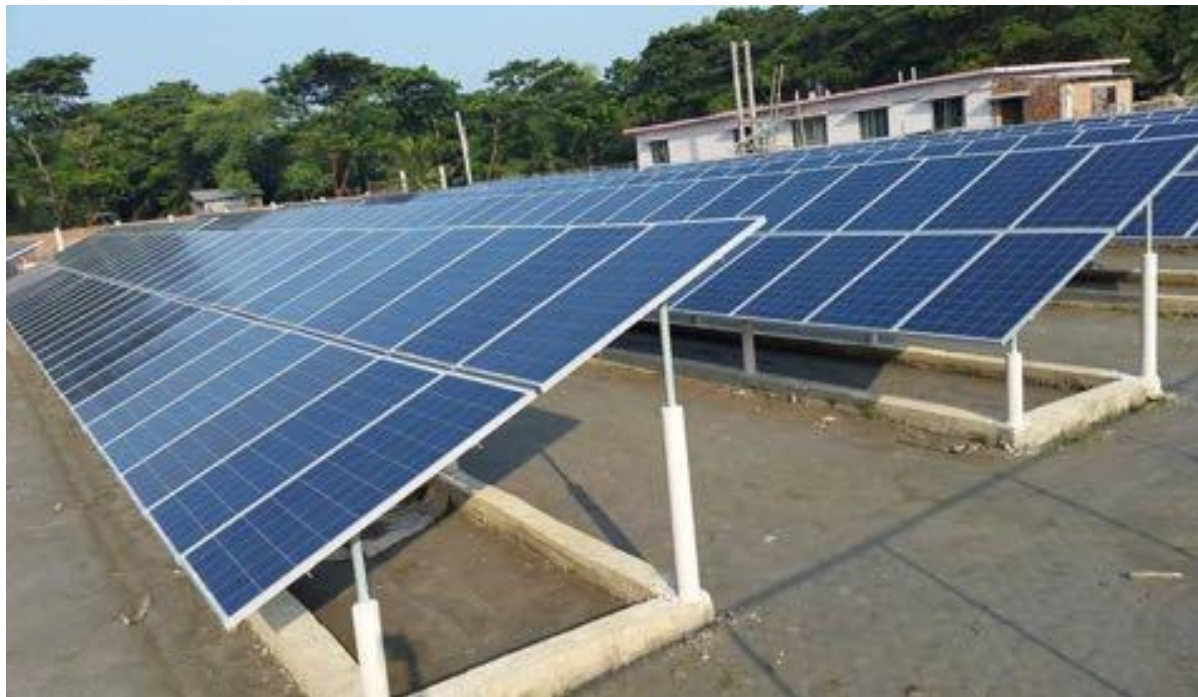
Example of beam type foundation
