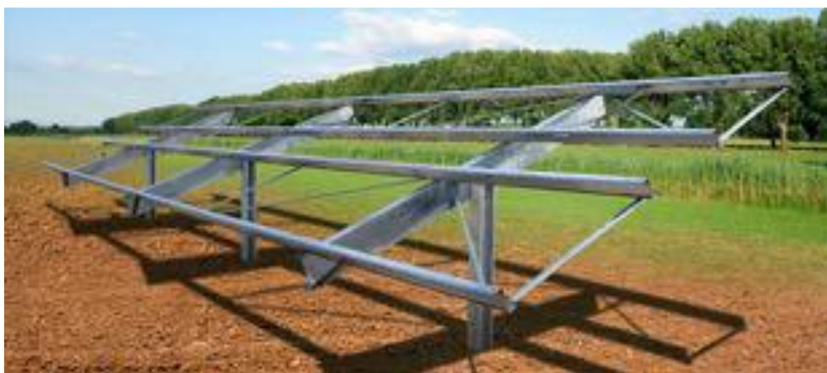
Example of pile foundation
