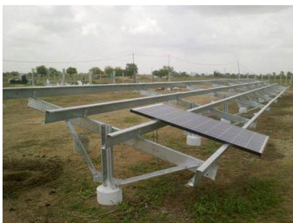
Example of block type foundation
