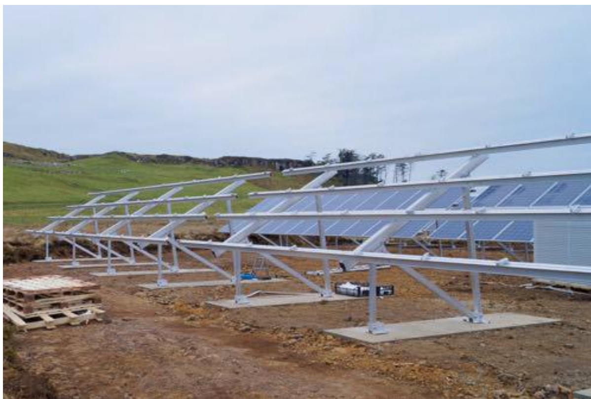
Example of slab foundation
