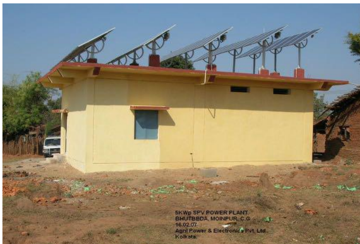
Example of array installed on a RCC roof of the control room
