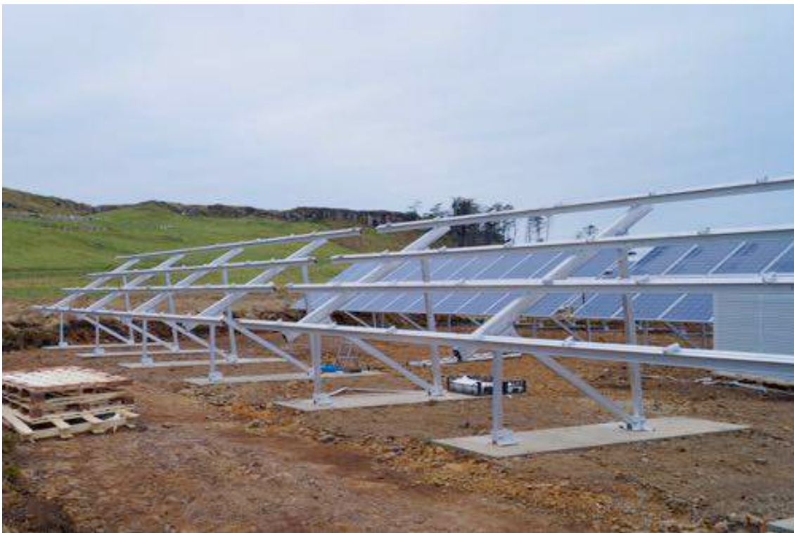
Example of slab foundation
