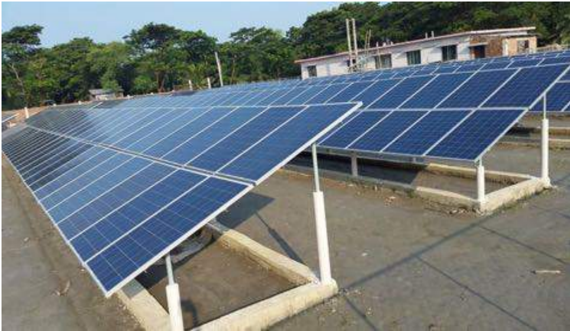
Example of beam type foundation
