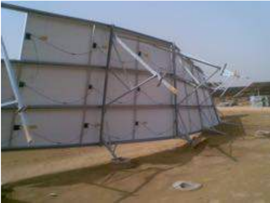
Poor quality structure and foundation
