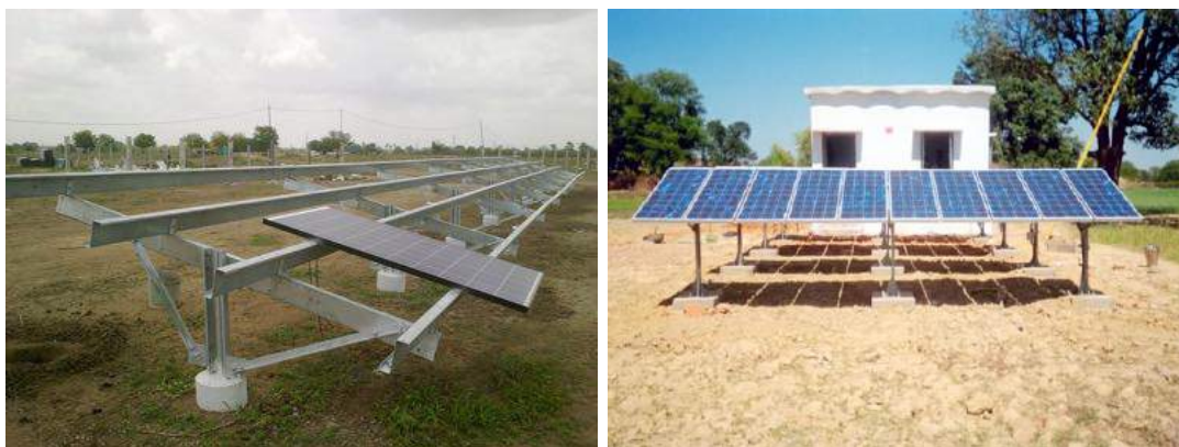
Example of block type foundation
