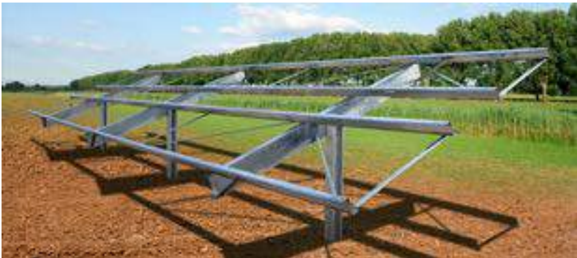
Example of pile foundation
