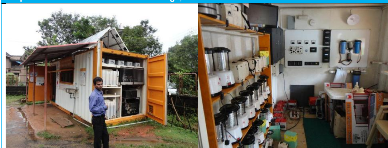
Photos 2.1 & 2.2: The exterior and interior views of a solar energy kiosk renting solar-charged lamps and batteries in Dharmasthala village, Karnataka
