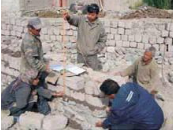
Construction of passive solar greenhouse at 14,000 feet
