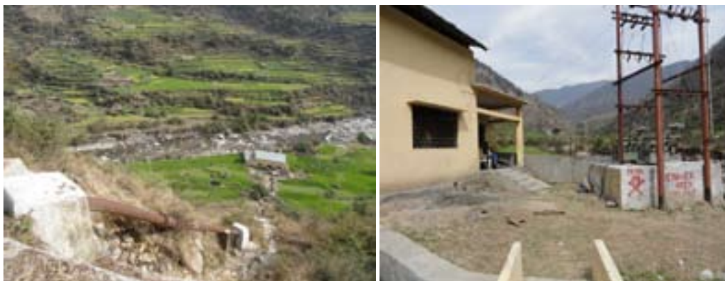
Jakhana micro hydel project, capacity 2 x 50 kW in District Tehri Garhwal of Uttarakhand
