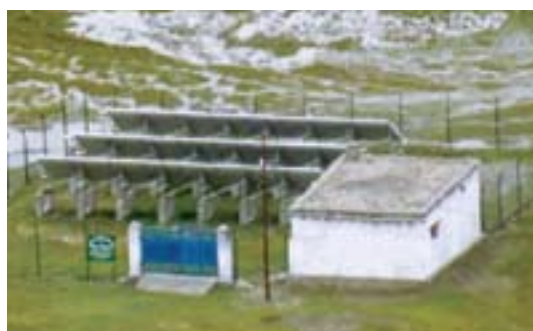
Solar photovoltaic power plant at Juldo
