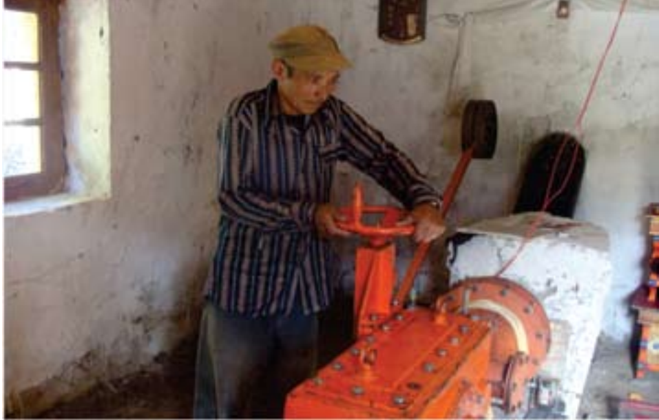
Udmaroo micro-hydro power unit
