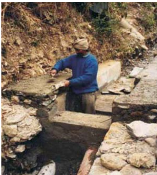
Construction of flow channel for watermill unit
